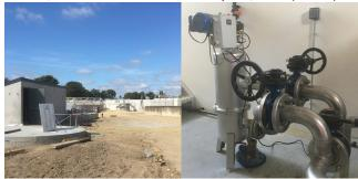
Filtration fer a wastewater clarifier-settler, before lagooning. Filter AG200 2" in 400  $\mu m.$
